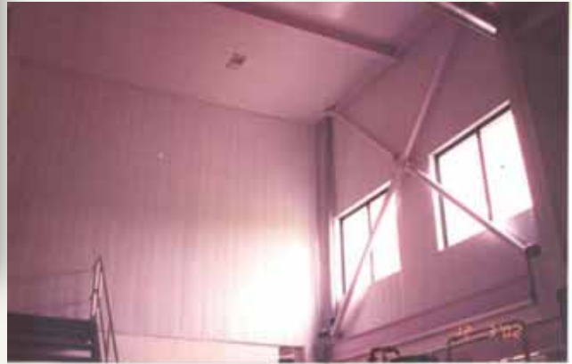
Cross Bracings and Partitions / Roof Liner
