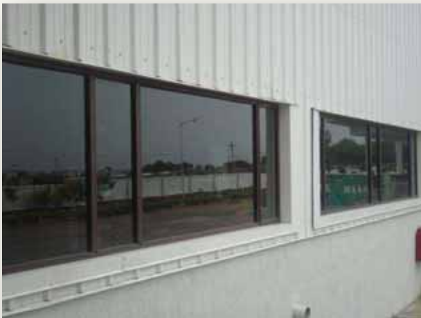
Framed openings for windows
